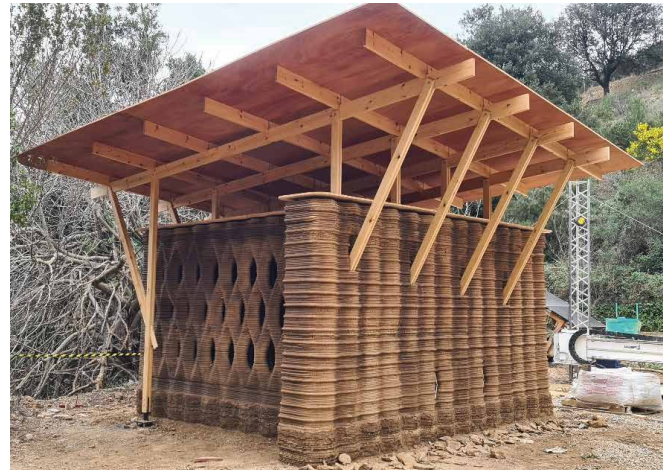
Figure 11: The 3DP earthen unit in Spain, at IAAC, 3DPA Program 21/22, Photo by Deena El-Mahdy, 2022
